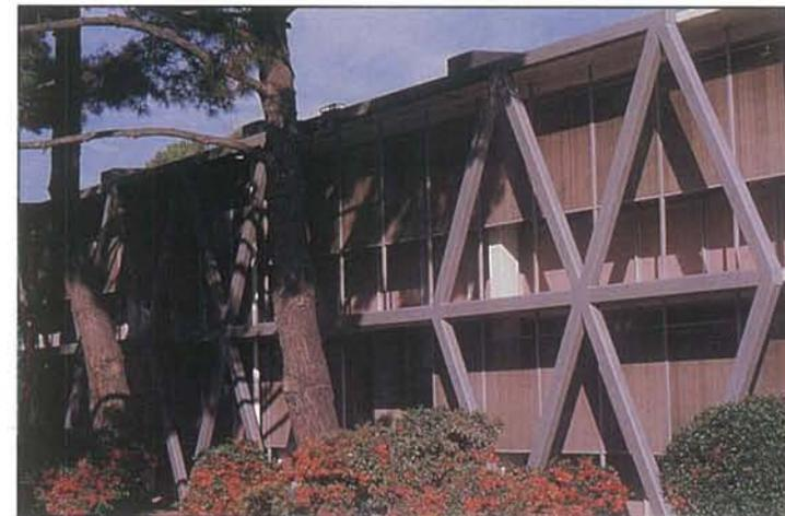
This diagonal steel frame effectively braces a concrete frame building housing U.S. Geological Survey employees.
