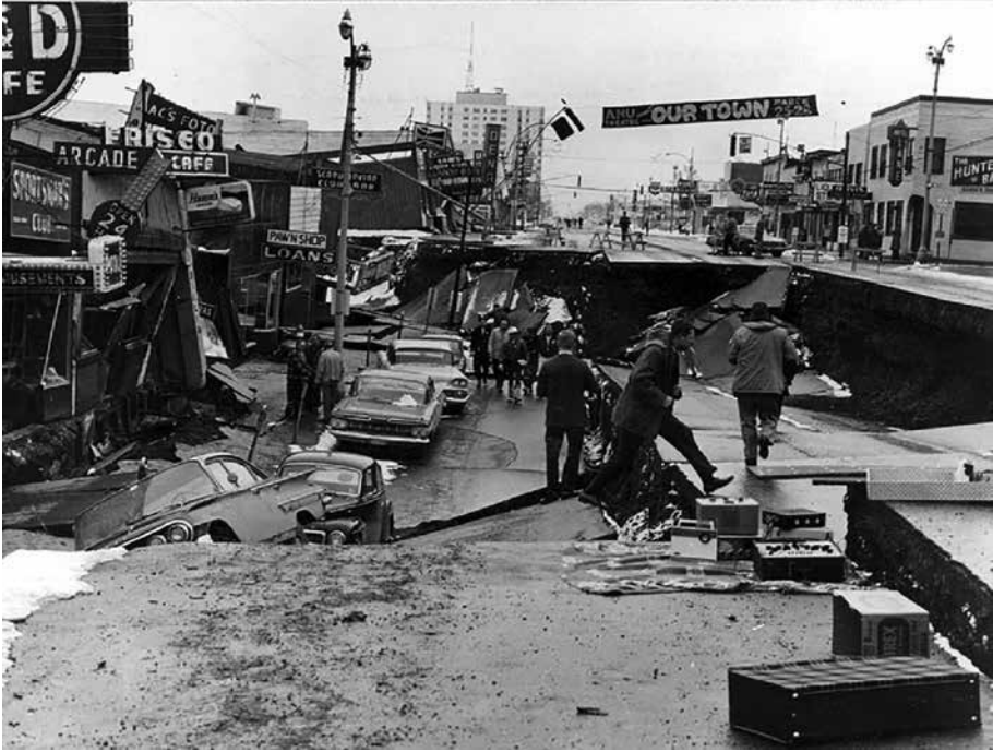
Figure 1.7 Five blocks along the north side of Fourth Avenue in Anchorage, Alaska, settled more than 12 feet during the Great Alaskan Earthquake of 1964.
