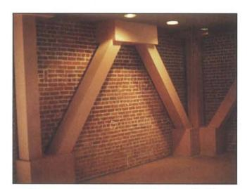
Unreinforced brick buildings pose a particular hazard even in moderate earthquakes. Unbraced parapets and walls inadequately tied to the floors and roof can topple onto sidewalks or adjacent buildings. Many such buildings are currently used for low-income housing and commercial space in the Bay Area. The Unreinforced Masonry Building Law required all local governments to conduct an inventory of
